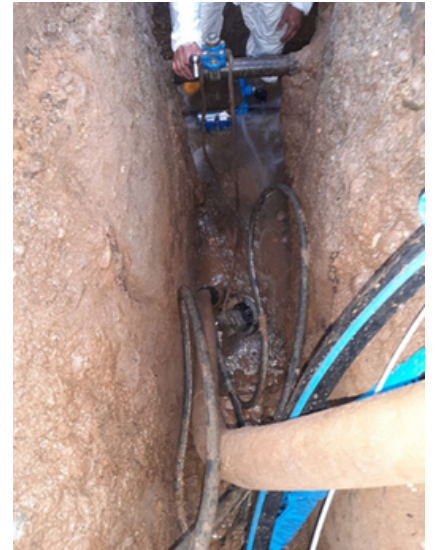
Figure 2 (above). Examples of quiet leaks in the water distribution network in the territory managed by Alfa S.r.l. detected via satellite analysis in collaboration with 2f Water Venture and ASTERRA.
