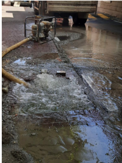
Figure 2 (above). Examples of quiet leaks in the water distribution network in the territory managed by Alfa S.r.l. detected via satellite analysis in collaboration with 2f Water Venture and ASTERRA.
