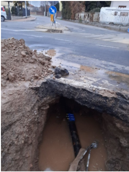
Figure 2 (above). Examples of quiet leaks in the water distribution network in the territory managed by Alfa S.r.l. detected via satellite analysis in collaboration with 2f Water Venture and ASTERRA.
